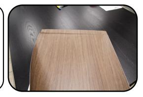
Slide your hand under the Wrap MK, gradually remove the protective paper from the adhesive. Glide the felt squeegee across the surface to eliminate air bubbles.
