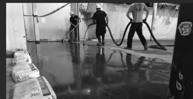
Level Set 200 pump application / Coulé de l'autolissant Level Set 200
